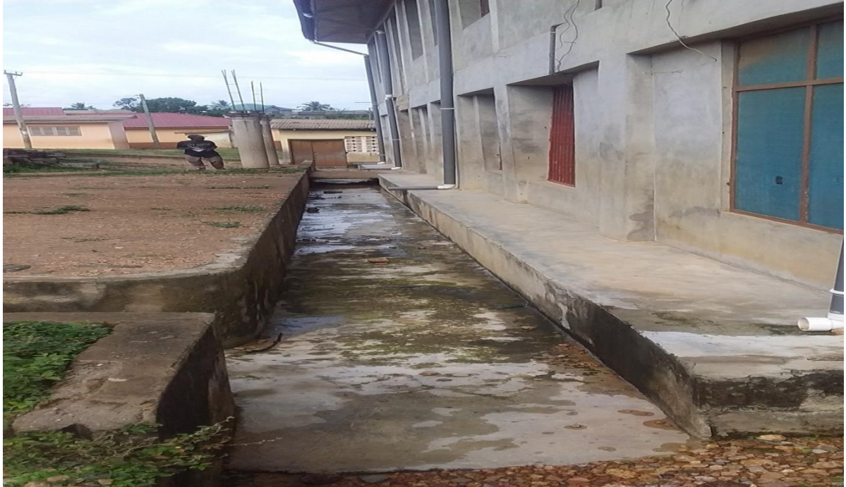
Fig P (This Uncovered gutter was identified at the Western side of the Woraba Church SDA Church Premises at Agona Swedru. PHOTO by: Ransford Osafo Gyasi on 13-10-2020 at 2:12pm).
