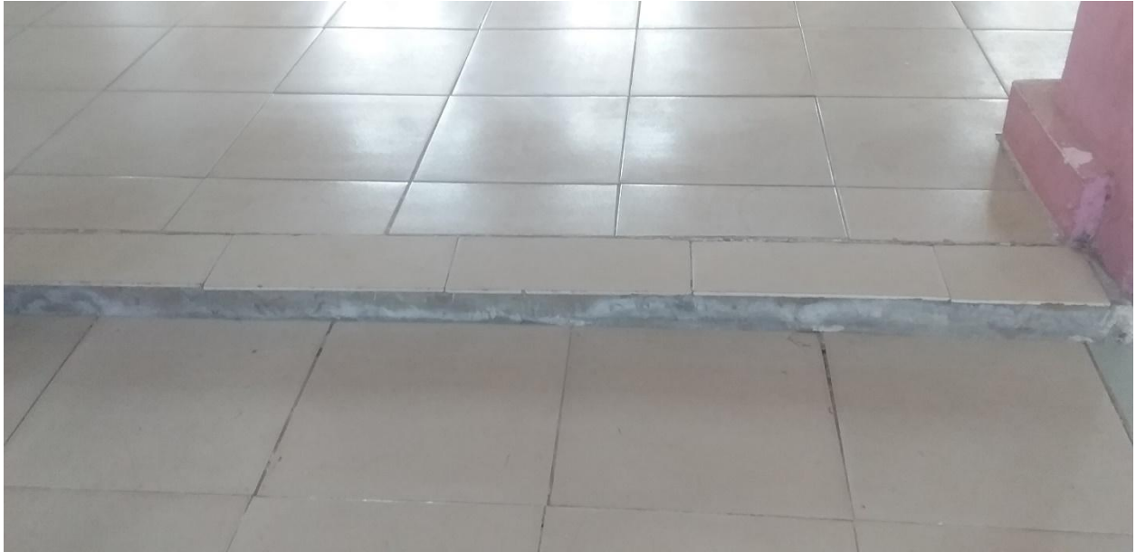
Fig J (An uneven floor found inside the chapel of the Winneba Church premises. PHOTO By: Ransford Osafo Gyasi on 13 th October, 2020 at 12:20pm).
